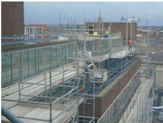
Window replacement programme
